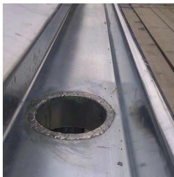
Downpipe outlet starter soldered to gutter
