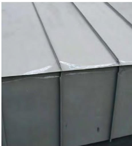
Staining resulting from partial removal of protective film.
